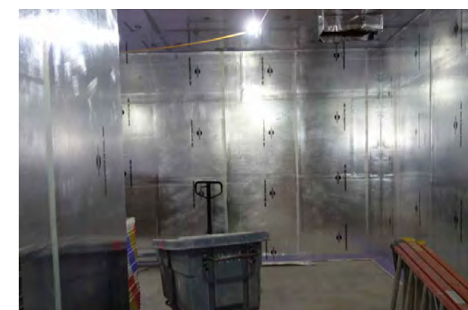
rFoil is installed on the walls of a new facility to meet complex building requirements.
