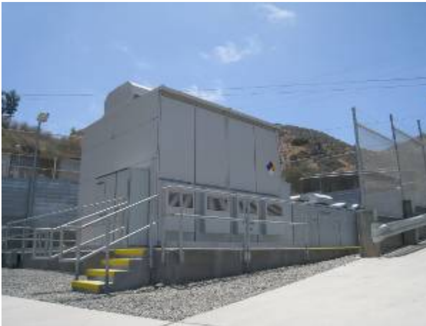
1MW/7.2MWh NAS ® Battery system at Catalina Island (SCE Pebbly Beach Generating Station)
