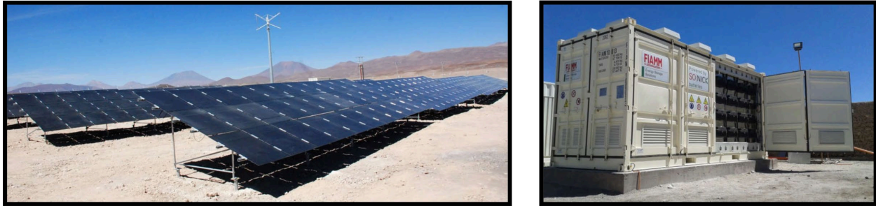
Figure 7. An FZSoNick Na-NiCl 2 battery system supporting integration of renewable remote photovoltaic energy in South America. Reprinted with permission of FZSoNick.
