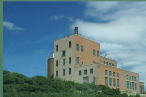
Raton Power Plant
