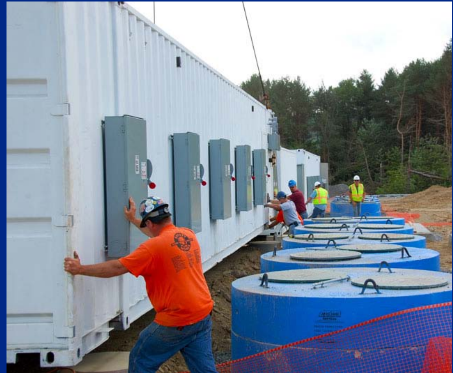
Construction of 20 MW plant in Stephentown, NY
