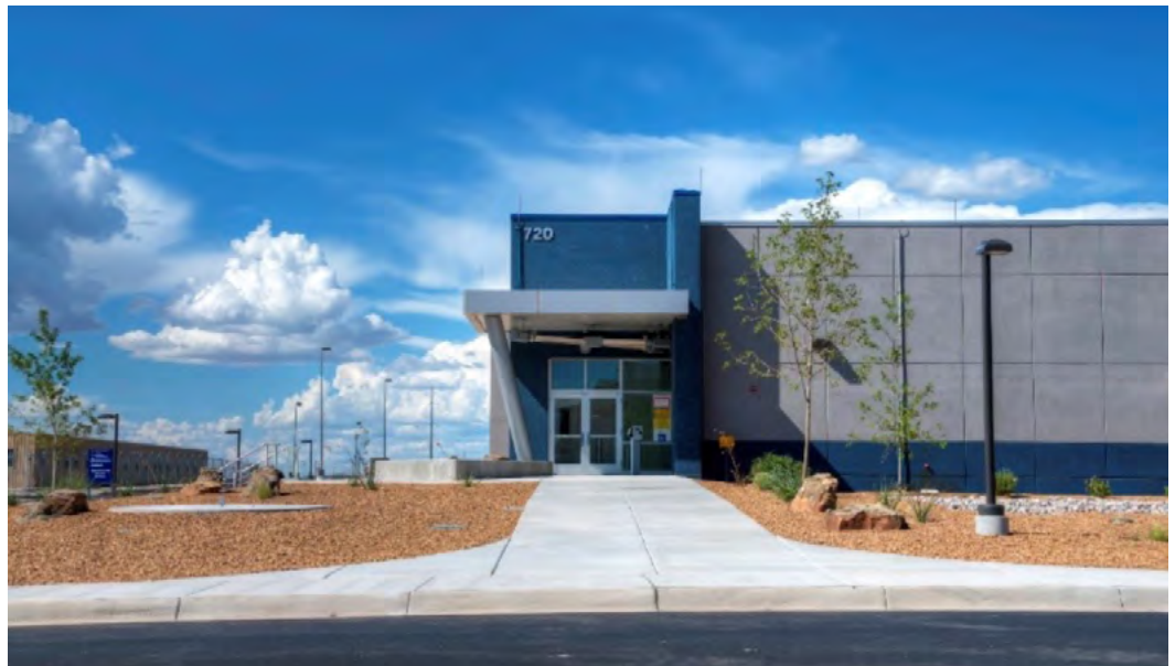
ICONIC ARCHITECTURE — The Ion Beam Laboratory was the first Sandia lab to earn LEED Gold status. Photo by Darrick Hurst
