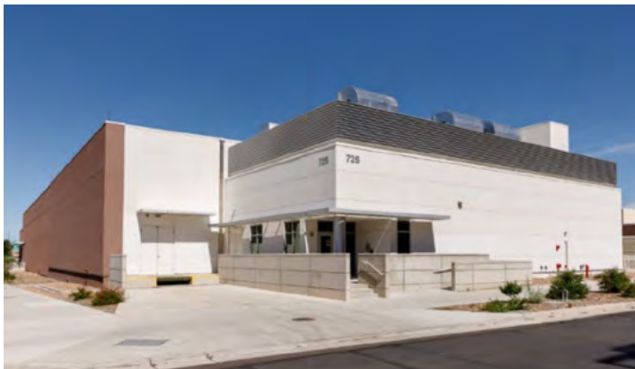
ASTRA-NOMICAL SUCCESS — Building 725E, home to the Astra supercomputer, earned a DOE Sustainability Award in 2020 for environmental efficiency. Photo by Bret Latter
