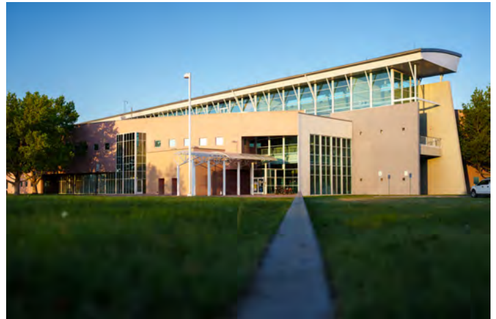
ROBOTIC MANUFACTURING SCIENCE AND ENGINEERING LABORATORY — Building 895, built in 1996, signifies Sandia’s shift in architectural ideology as it sought to have buildings reflect innovation in science and technology. Photo by Craig Fritz
