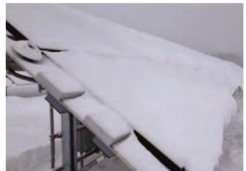
SNOWBOUND — Snow cover on photovoltaic systems can block light and create ice dams, resulting in significant power losses and reliability concerns. Photo by Laurie Burnham
