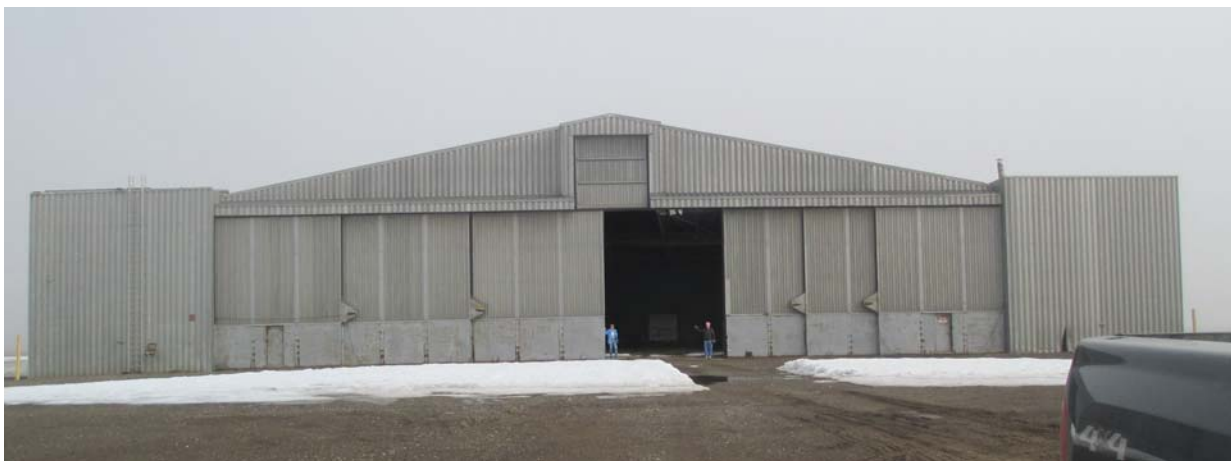
BIG PLACE IN A BIG SPACE — Jerry Peace, left, and Mark Ivey offer size perspective to an abandoned Air Force hangar only a few hundred yards from the Arctic Ocean at Oliktok Point. Mark is negotiating with a private company in Deadhorse, located at the beginning of the peninsula, for a hangar fall-back if complexities make use of the Air Force hangar too difficult.
