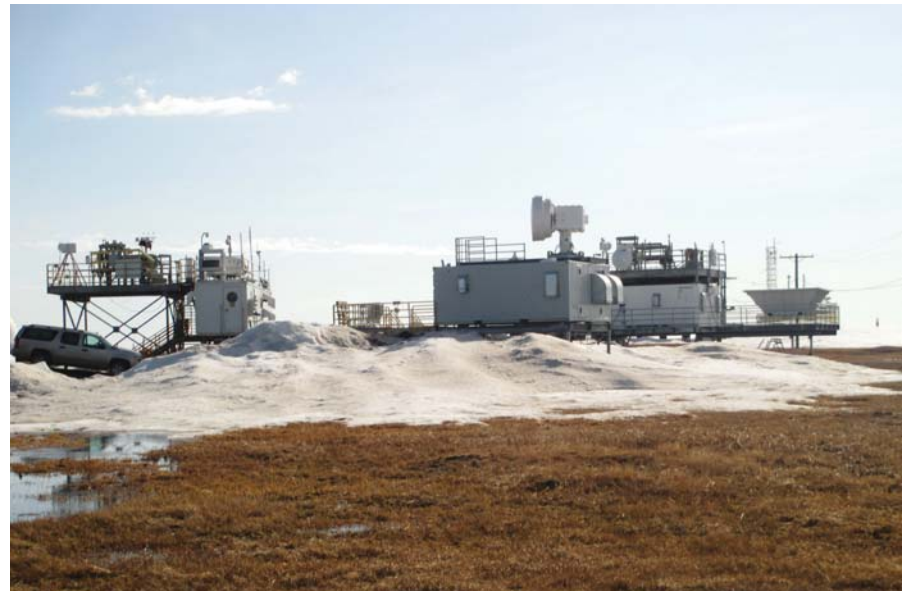
INSTRUMENT SHELTERS and new radar are part of the ARM facility near Barrow.
