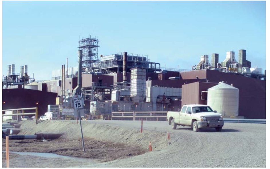
ONE OF THE GIANT OIL processing plants bordering Prudhoe Bay. Although fewer than 2,200 people live in the region permanently, several thousand transient workers support the area's oil fields.
