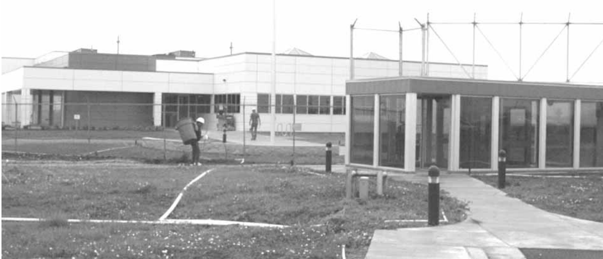
CONSTRUCTION WORKERS put finishing touches on the new WETL building.
