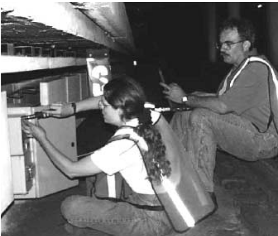
BETH WICHMAN (8222) and Ray Trechter (9522) install prototype chemical early-warning system detectors in the Washington Metro in July 2000.
