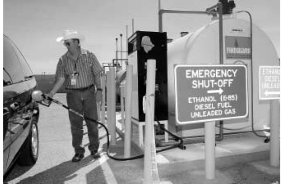
PUMPING ETHANOL — Chuck Kearns of Sandia's Fleet Services Dept. 10849 pumps E-85, a new alternative fuel, into one of Sandia's "flex-fueled" vehicles. These vehicles can operate on E-85, which is a mixture of 85 percent ethanol with unleaded gasoline, or traditional fuels. Sandia's motor pool fueling station also offers bio-diesel and compressed natural gas fuels. (Photo by Randy Montoya)
