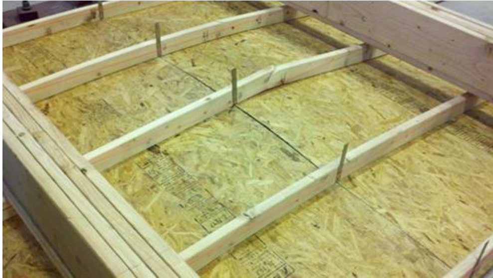
Figure 25. Typical failure in rafter, most occurred in center.
