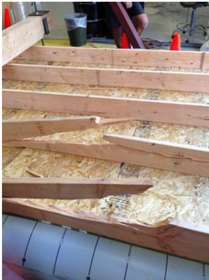
Figure 26. Failure in rafter, some occurred in side rafters.
