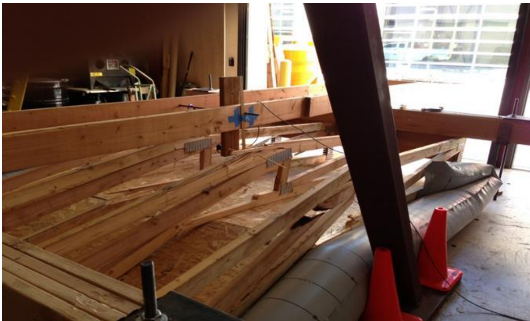
Figure 28. Failure in open web (member connection) truss roof test assembly.
