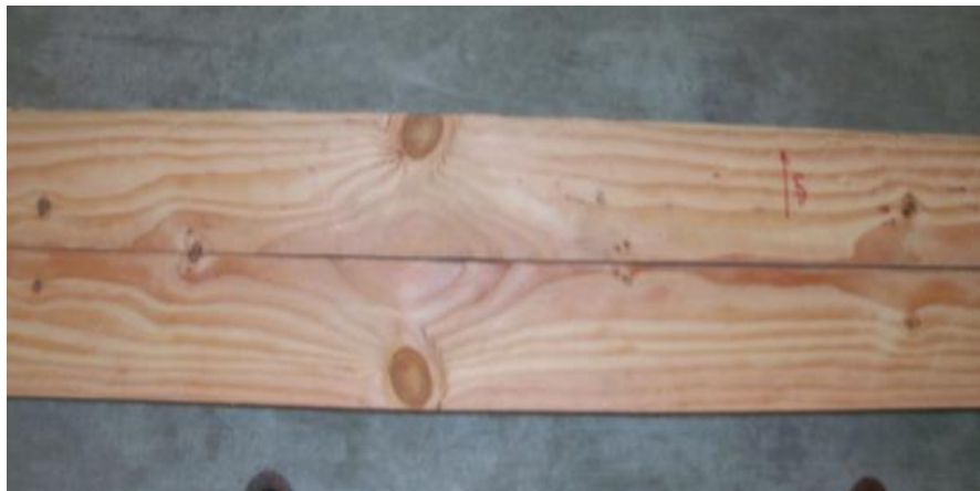
Figure 8. Twin 2"×4" joists cut from a single 4"×4" joist.
