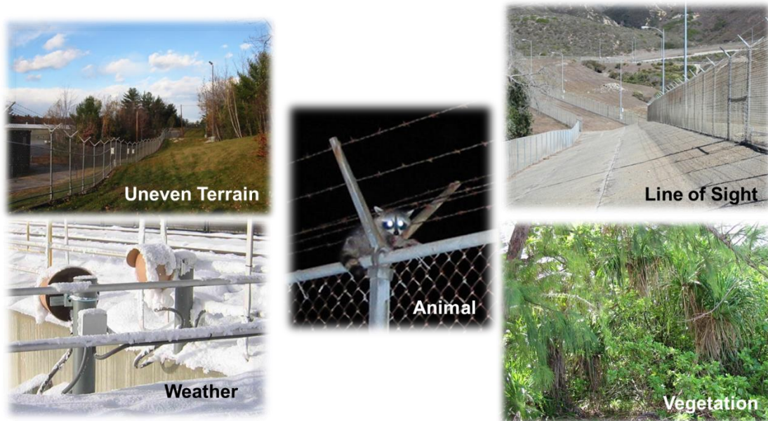
Figure 5. Conditions that Affect Exterior Sensors
