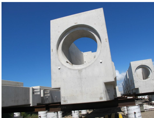
Figure 3-23. AHSMs base units at SONGS.
