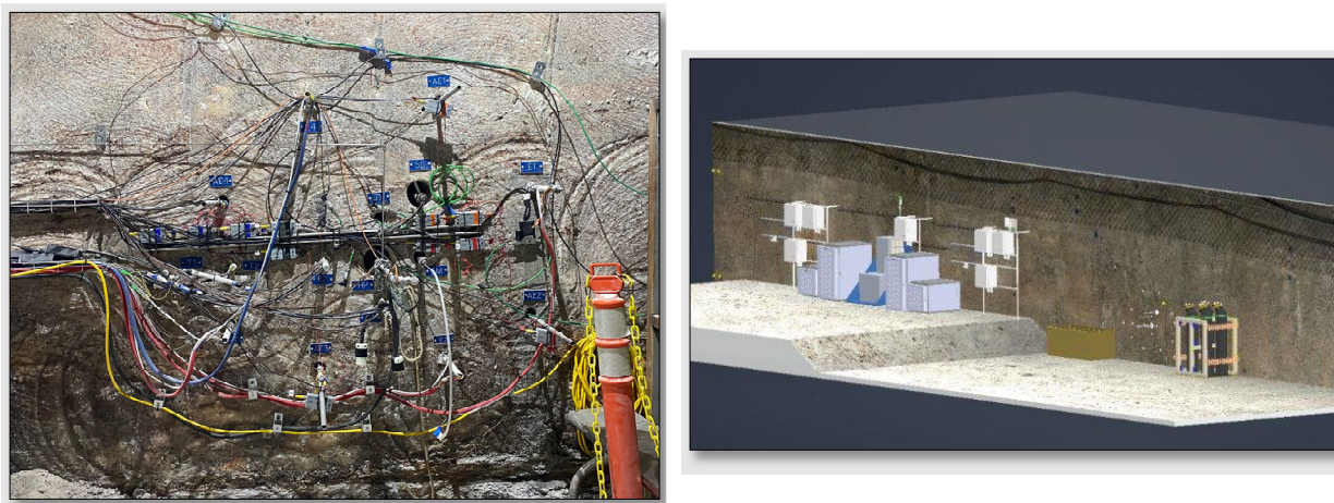
Figure 2-2. BATS Phase 2; photo of BATS 2 array (left), and layout of in-drift equipment (right).
