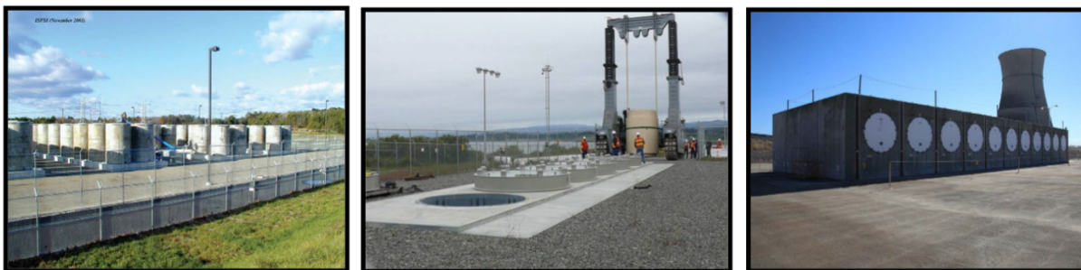
(a) Vertical Above Ground (Maine Yankee, Wiscasset, ME)
