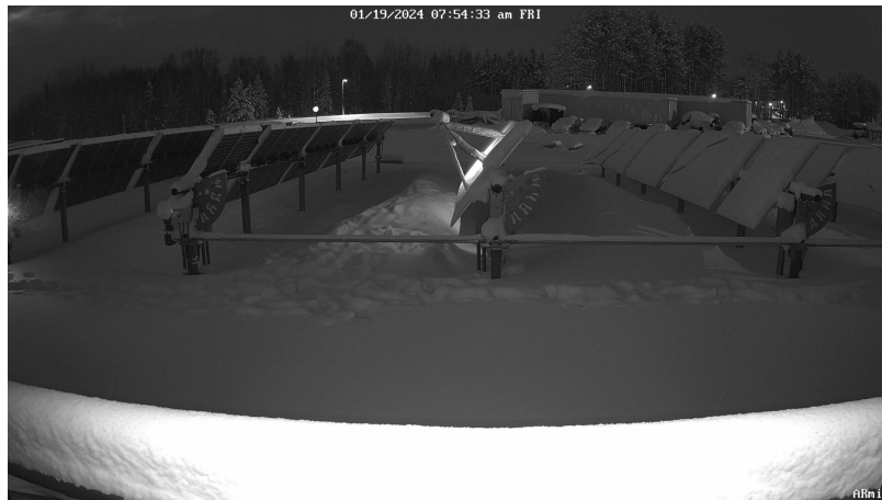
Snow shedding even observed on 19 th January when the panels were at maximum tilt
