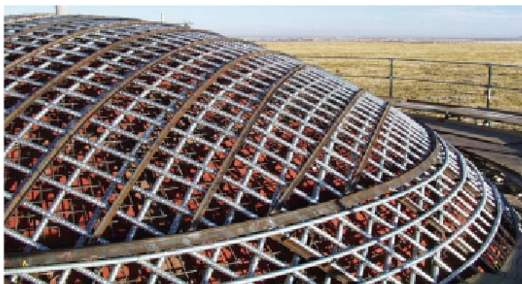
Figure 3.2 Arrangement of tendons in the dome.
