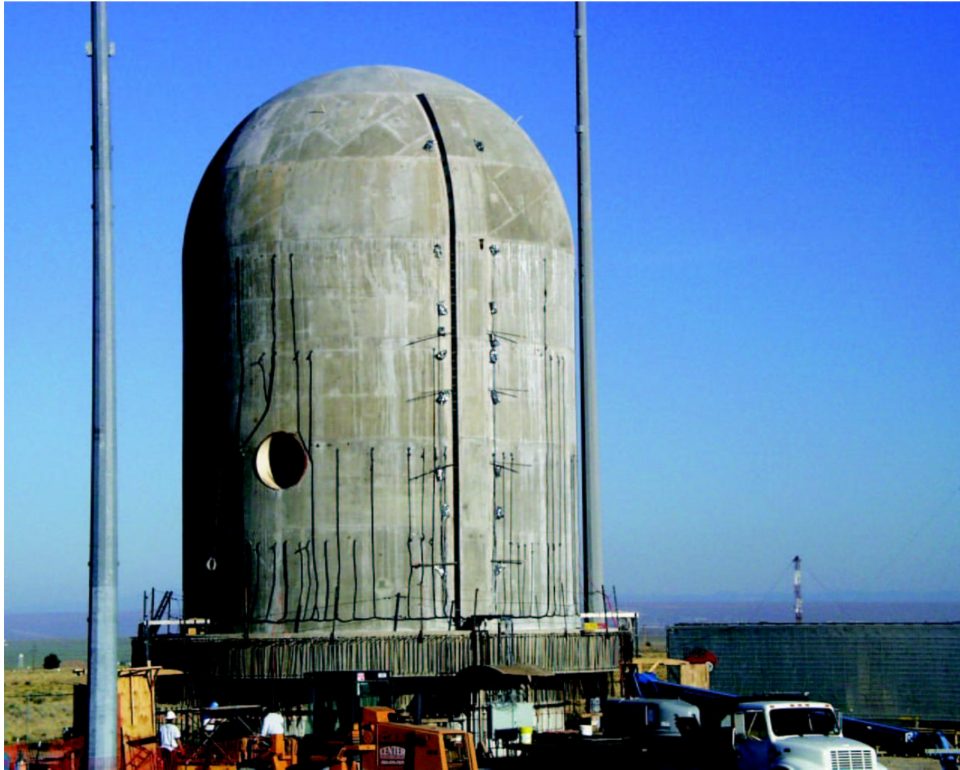
Figure 1. NUPEC/NRC 1:4 Scale PCCV Model Built at Sandia National Laboratories
