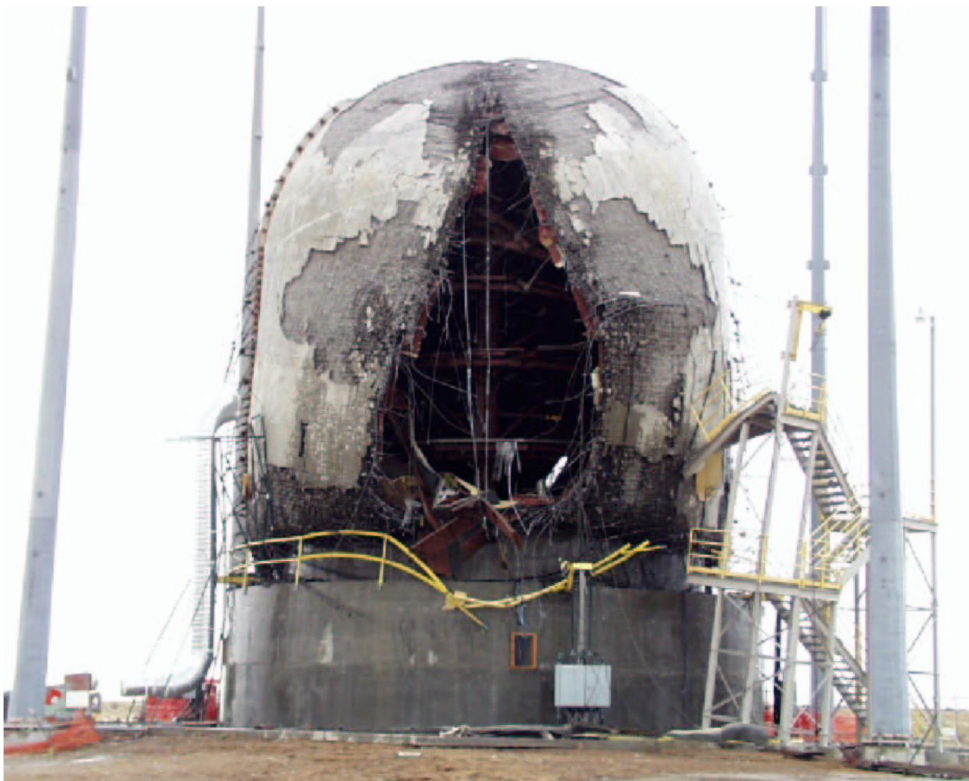
Figure 3. PCCV Model after Structural Failure Mode Test
