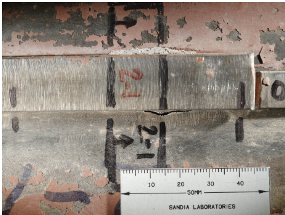
Figure 50. Details of inside (top) and outside (bottom) liner features in region of tear #2-1 metallographic cross-section (arrows begin at plane of section and indicate view direction).
