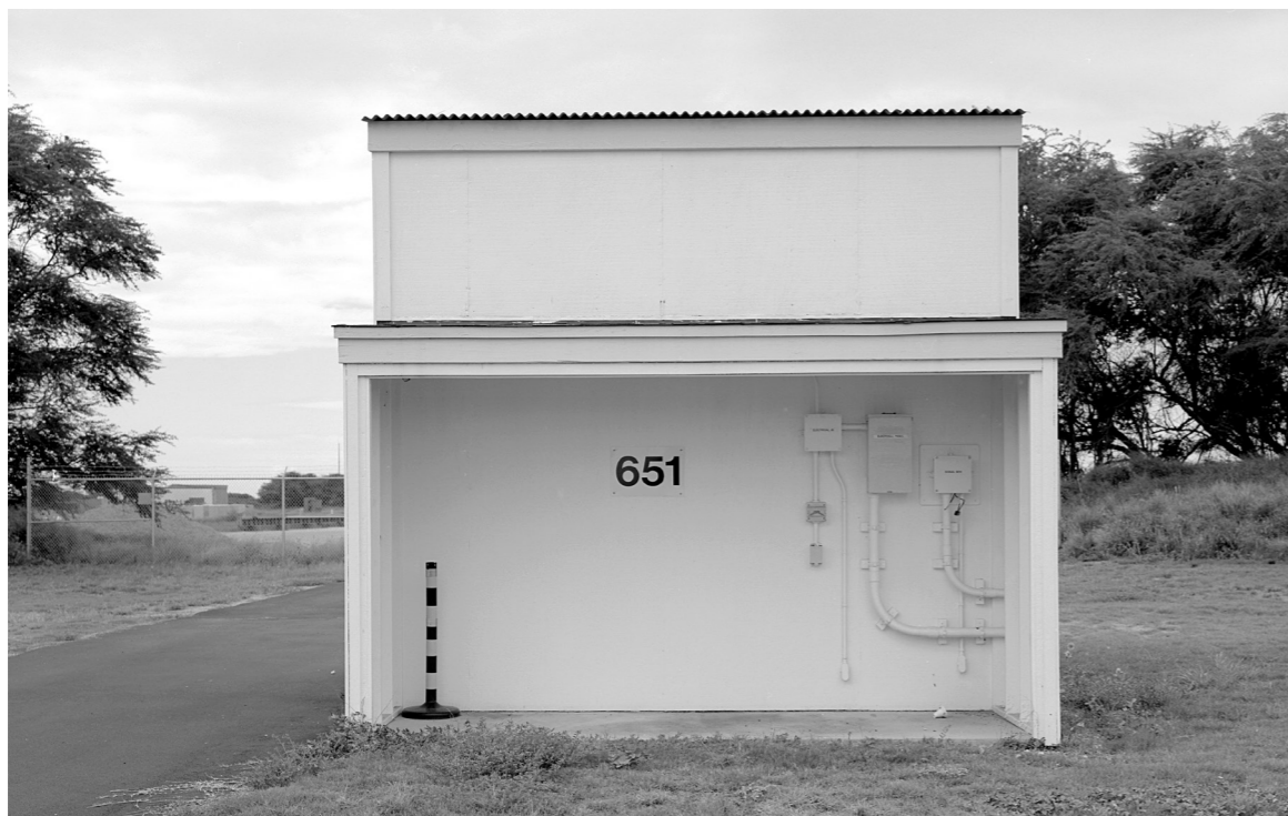
Building K651, Balloon Release Building, 2006 (photographer Joseph Bonaguidi)
