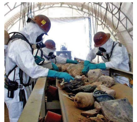
Technicians sort waste excavated from Sandia's chemical waste landfill.
