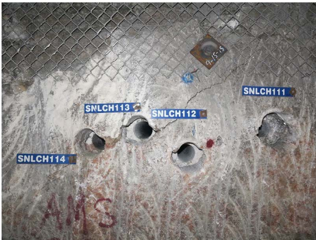
Figure 24: Picture of boreholes used to collect brine samples for analysis. Boreholes are located at the SDI experimental area at WIPP.
