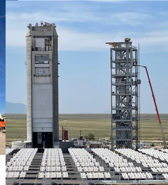
Tower Complete Solar Equipment Loaded Commissioning underway Today
