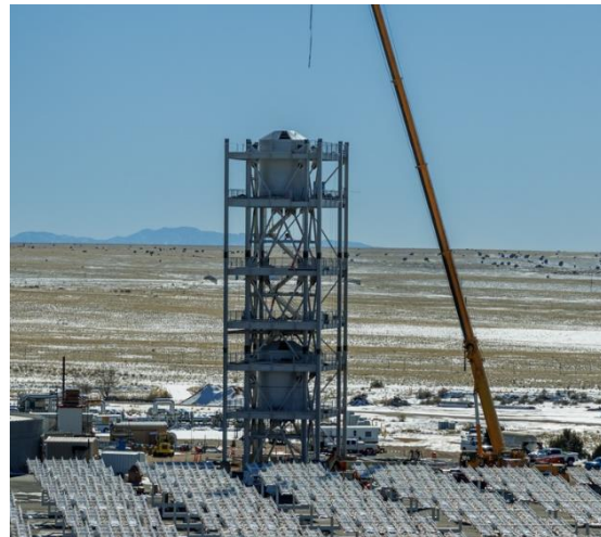
Completed installation of hot storage bin
