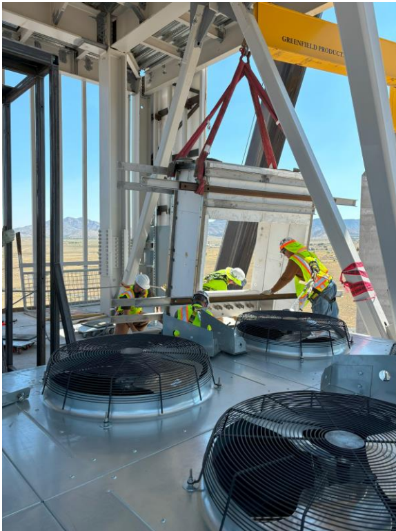
Receiver cavity being lifted into the tower
