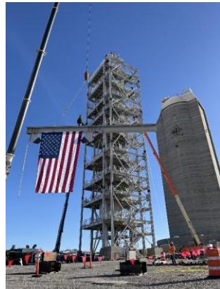
Tower top out
