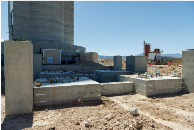
Poured and cured drilled piers and pier caps
