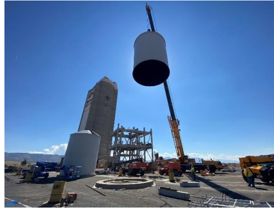
Installing "cold" storage bin
